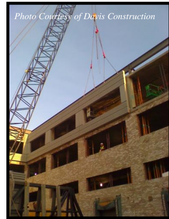
Figure 5 | Precast Panel Installation
