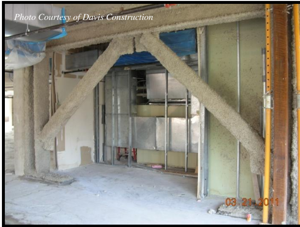
Figure 4 | Installed Seismic Bracing
